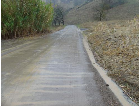
Compacted road surface draining water to ditch
